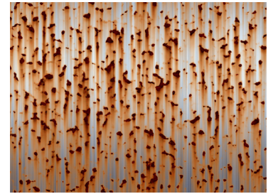
Unacceptable rusty surface
